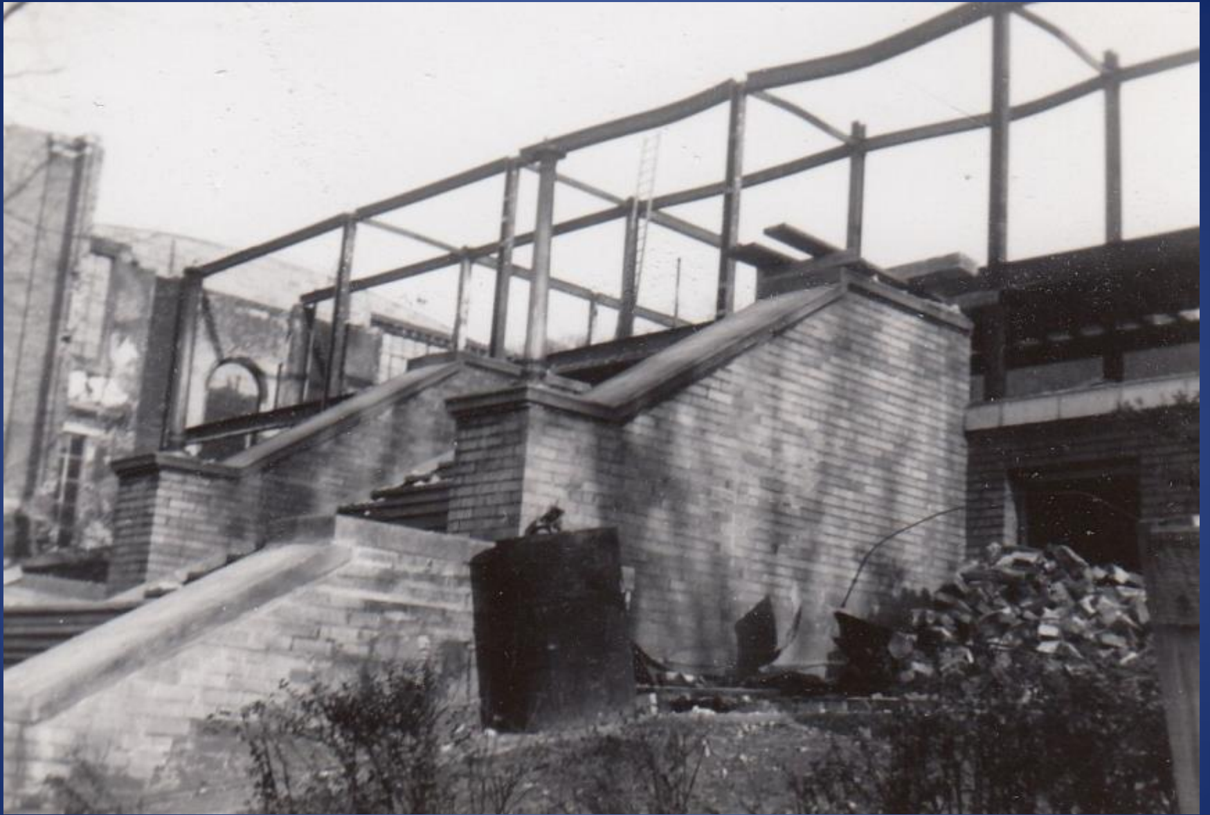
Results of Hinton High School Fire Main Entrance
