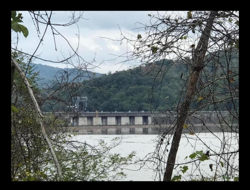
The spillway on the lower side of the dam is only functioning at half capacity, due to the long-term construction project.
